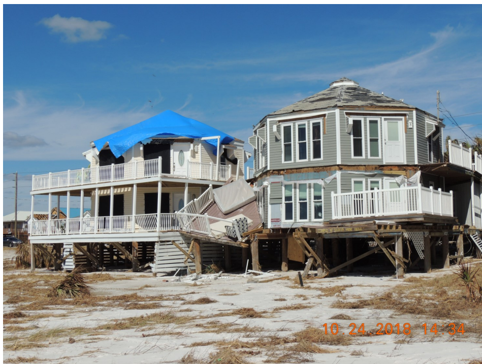
Two surviving structures that are potentially substantially damaged on the Gulf beachfront at Mexico Beach.
